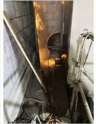
HF Wall Sawing
