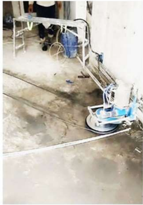
HF Wall Saw Cut Steel Rebar
