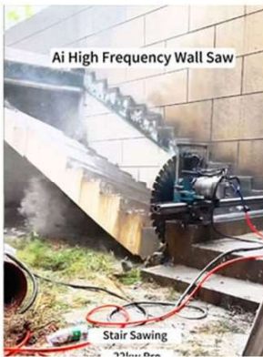
Dua Use of High Frequency Wall Saw
