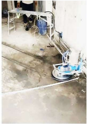
HF Wall Saw Cut Steel Rebar
