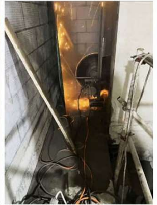
HF Wall Sawing
