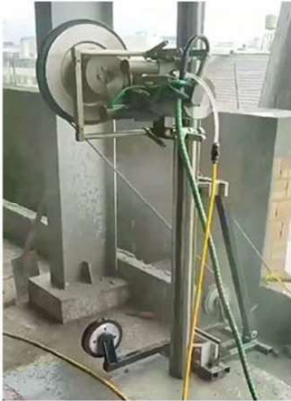
Wire Saw Head Unit with High Frequency Motor
