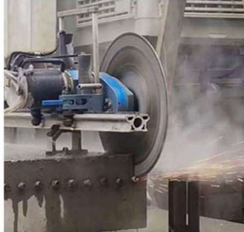
HF Wall Saw Cut Steel Rebar
