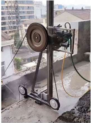
Wire Saw Head Unit with High Frequency Motor
